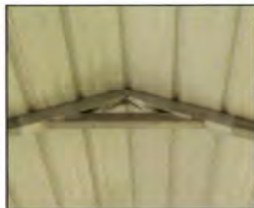
Welded Supports on all Building 20' and Wider
