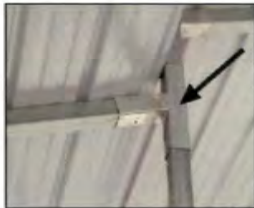
Stronger Construction (Barns Welded Supports)
